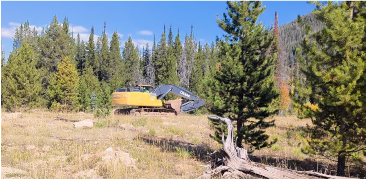
Figure 2 - Excavator on Thunder Mountain Road
